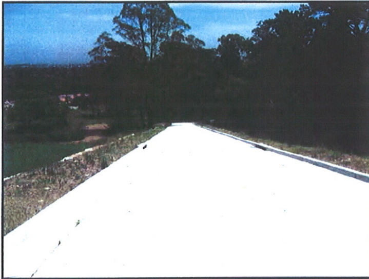
View looking west from Old Northern Road of recently constructed access driveway.
