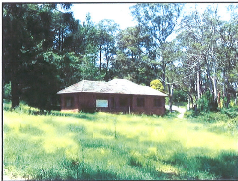
Subject property - View of existing residence.
